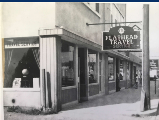
32 2nd St West Office
